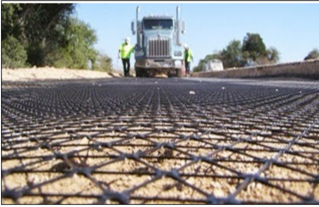
Fig. 2: Geogrids as soil reinforcement
